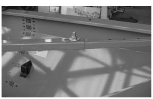
Figure 5.15: Fasten the centre part of the strut.
