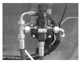
Fig. 22: Flow control valve
